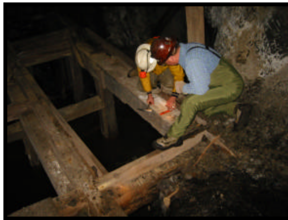
Figure 8. Installing Spad @ Bachelor Shaft
