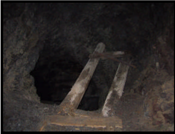
Figure 3. Bachelor Shaft Before Rehab
