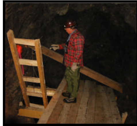
Figure 4. Bachelor Shaft After Rehab
