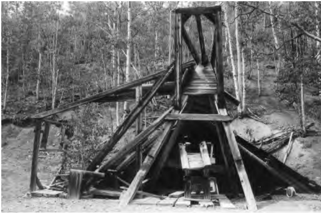
Figure 7.8 The photo depicts the south elevation of the shaft house standing over the Phoenix Shaft. The structure consists of corrugated iron siding nailed to the headframe (Feature 3) at center, an A-frame extending behind the headframe, and framing to the left. The framing enclosed the hoist, which was anchored to a timber foundation (Feature 4) that manifests as the bench-like structure. The timber structure underneath the headframe upended an ore bucket, and directed the bucket's contents into a waiting ore car. The Outlet Mining Company built the structure in the 1950s. Source: Author.
