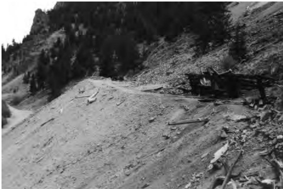
Figure 7.13 The photo is an east view of the Main Haulageway's surface plant remnant. The structure at right is the shop remnant (Feature 31), built around 1891. The tunnel portal (Feature 27) is adjacent and right. The aerial tram engine (Feature 35), installed during the 1940s, is visible near the end of the waste rock dump. East Willow Creek is visible at left. Source: Author.
