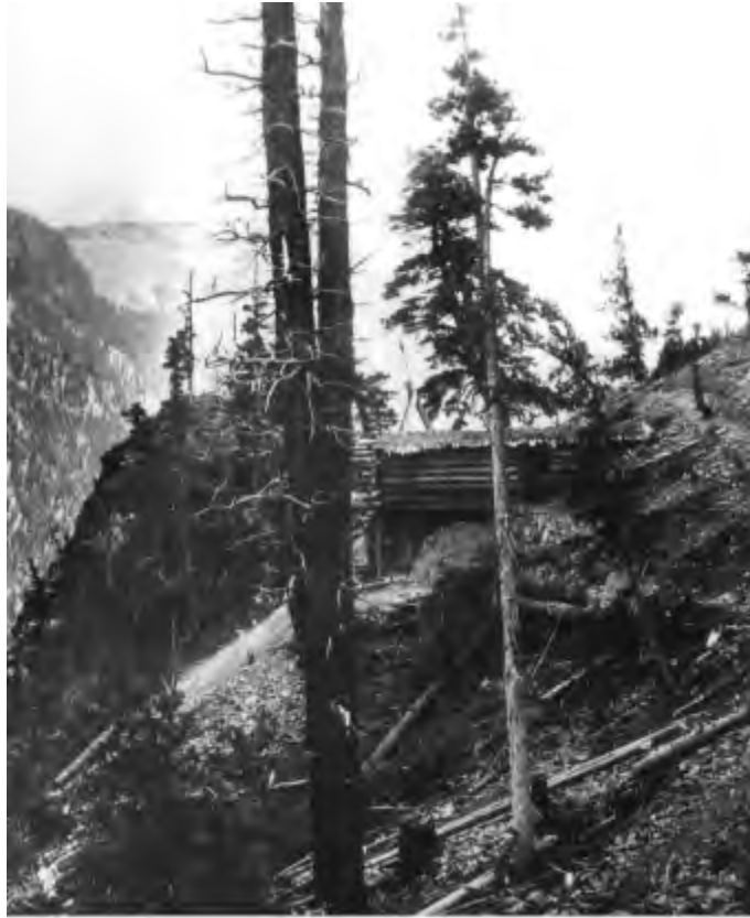
Figure 7.3 This south view depicts the log shaft house that stood over the Holy Moses' southern shaft. The right portion of the log structure stands over Feature 5 (Shaft House Platform), and the left portion stands over Feature 4 (Shaft House Remnant). The structure was erected around 1891. Note the tripod headframe extending out of the left portion of the roof. Courtesy of Colorado Historical Society.
