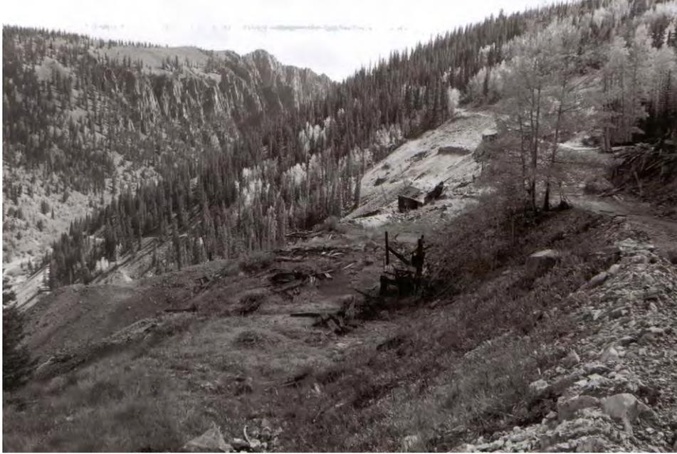
Figure 7.3 The remnant of the Amethyst Shaft's surface plant as it appears today. Compare this photo with the two upper views. The coal bin remnant (Feature 7) is right of center, and the ore sorting house erected during the 1910s (Feature 14) can be seen above center. Author.
