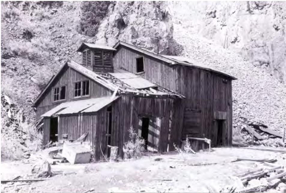
Figure 7.20 View north of the shop building (Feature 10). The building's left portion housed the blacksmith shop, the right portion housed a machine shop, and a change room occupied the second floor. Author.
