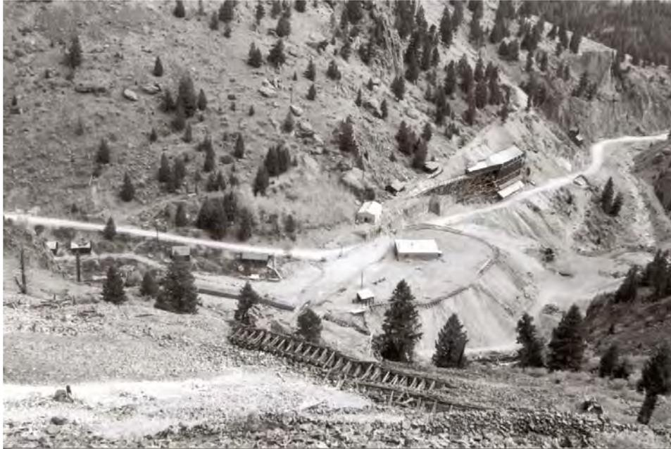
Figure 7.29 Overview down and east of the Commodore Tunnel No.5 complex. The Bachelor Loop road is visible passing through the site, and the cribbing wall retaining the Bachelor Mine's waste rock is at photo bottom. Author.
