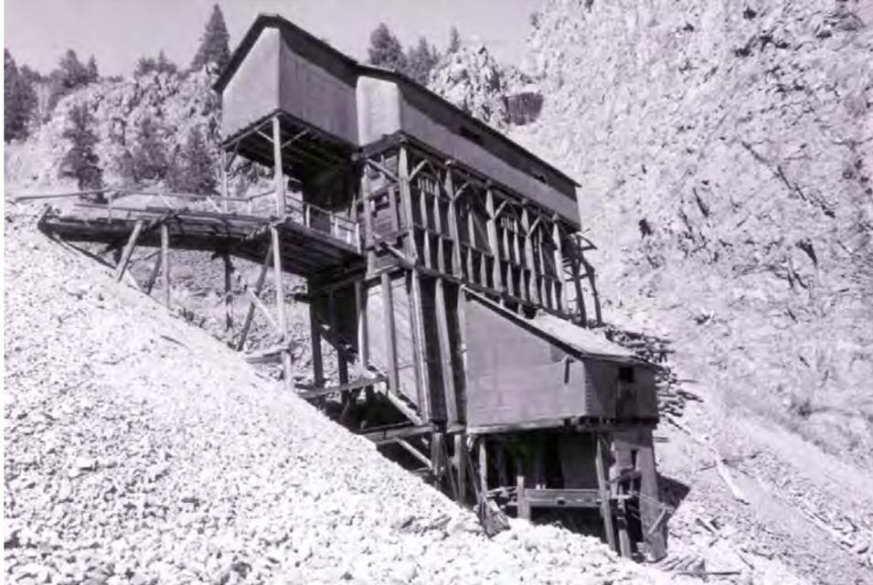
Figure 7.24 Quarter view up and west of the mine's ore sorting house and aerial tram terminal (Features 16 and 18). The tram terminal stands at the base of the ore sorting house.
