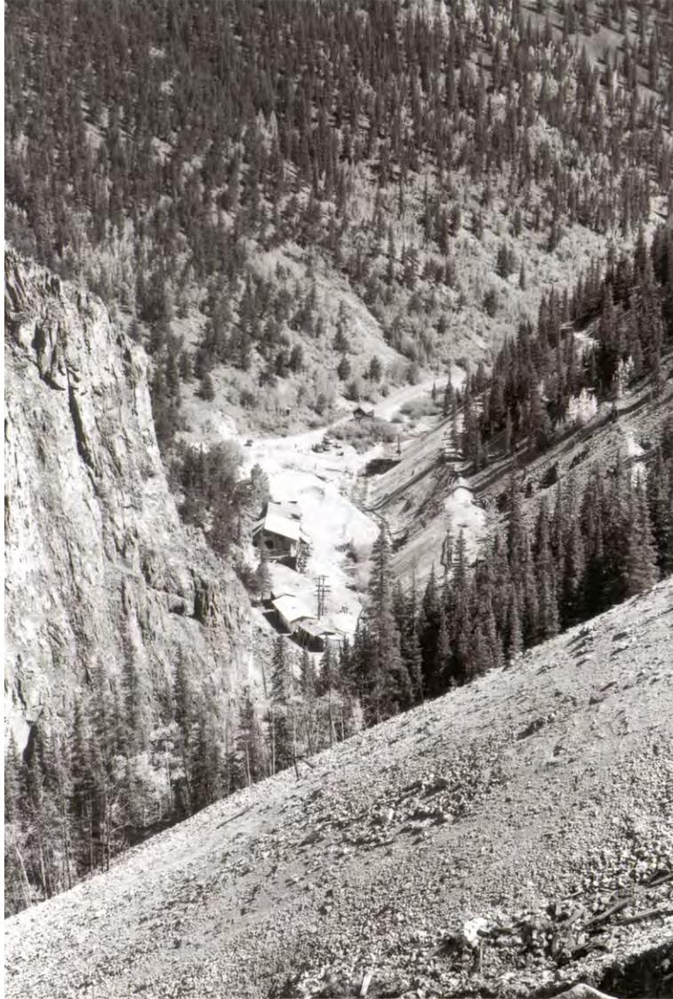
Figure 7.11 Overview east of the Amethyst Tunnel complex. The series of buildings near photo center consists of, top to bottom, the ore sorting house, the original compressor house, a new compressor house, and the barn (Features 16, 13, 12, and 11, respectively). West Willow Creek flows through the center of the photo, and waste rock dumps (Features 2 and 4) flank the creek. Bachelor Loop road traverses the photo above the buildings. Author.
