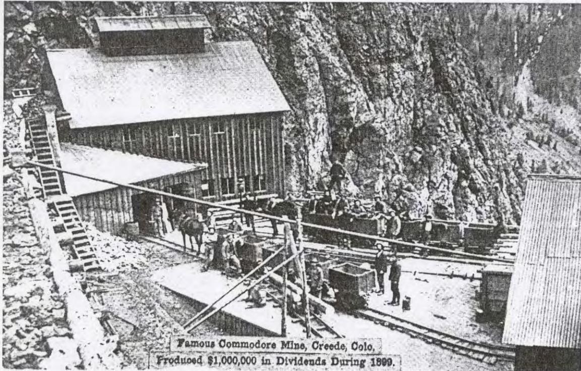
Figure 7.14 This late 1890s scene depicts miners and trains of empty cars at the entrance to the Bachelor Mine's upper tunnel. The large and complex building at left was the tunnel house and blacksmith shop. The building at right was probably a machine and carpentry shop. None of these structures remain today. Courtesy of Colorado Historical Society (S0025669).
