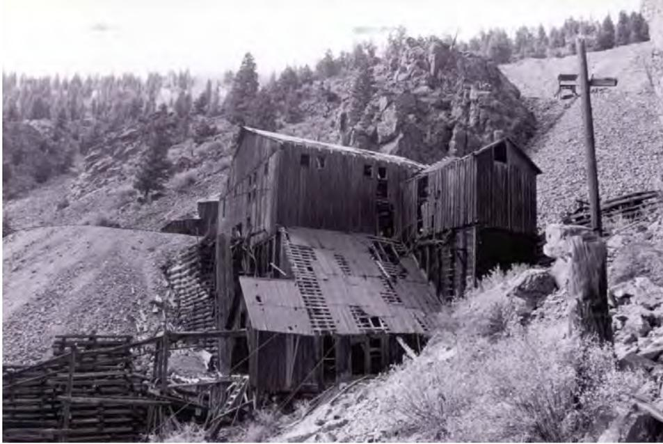
Figure 7.19 View southwest of the aerial tram terminal (Features 18 and 19). The terminal is the structure with the slanted roof, and the ore sorting house stands above. Tram buckets traveled up the timber beamwork at the lower left and into the terminal. Author.
