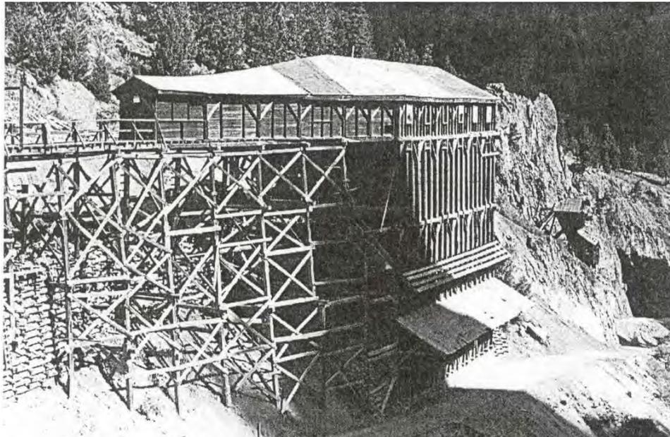
Figure 7.30 View east of the mine's two ore sorting houses. Feature 47 is the prominent structure, and Feature 57 clings to the cliff in the background. Author.
